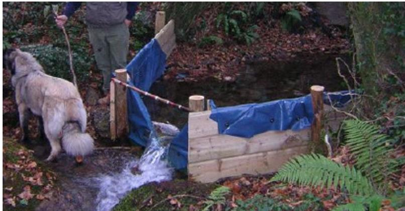
**Figure 3: Suggested method of V-notch weir construction**
