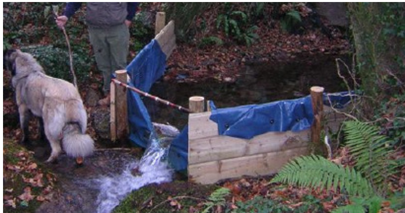
Figure 3: Suggested method of V-notch weir construction
